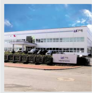
Dalian Plant (China)
