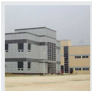
Wuxi Plant (China)
